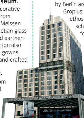
The station entrance on Potsdamer Platz.
